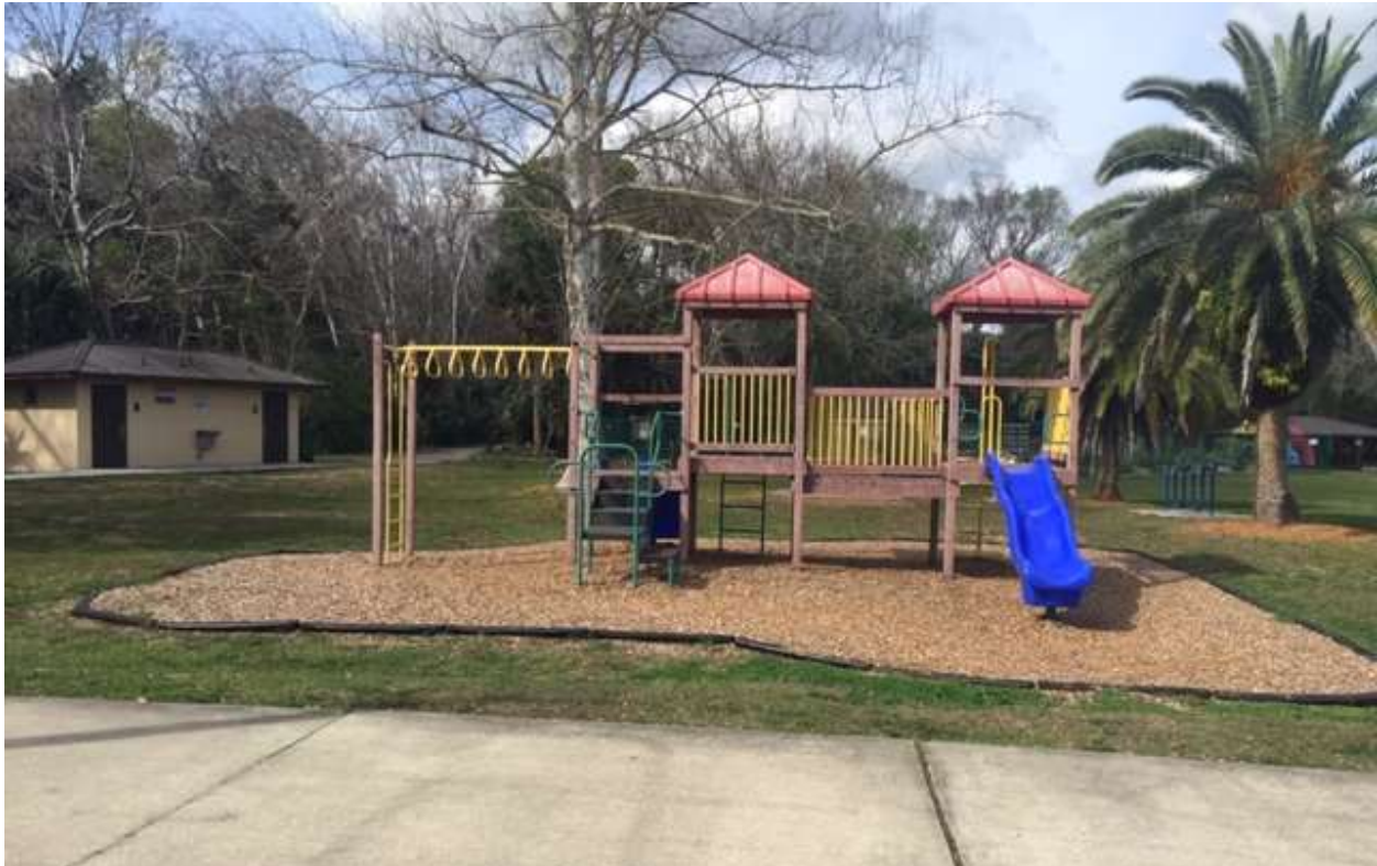
PHOTO LOOKING NORTH – SHOWING EXISTING SITE CONDITIONS/EQUIPMENT
