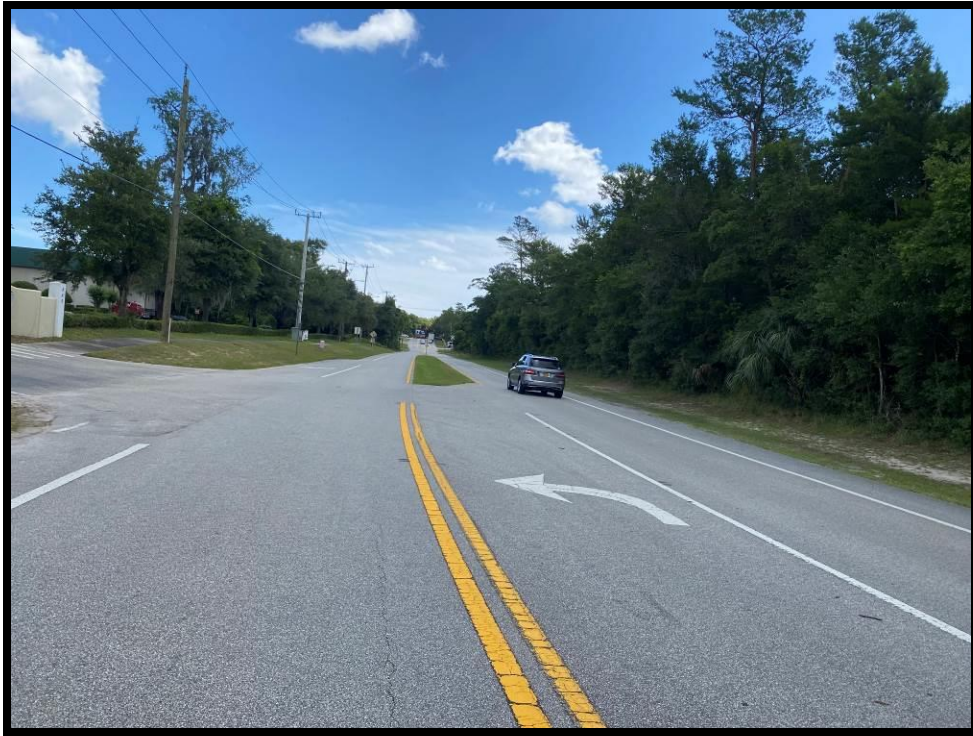
VIEW OF AIRPORT ROAD FACING WESTERLY
