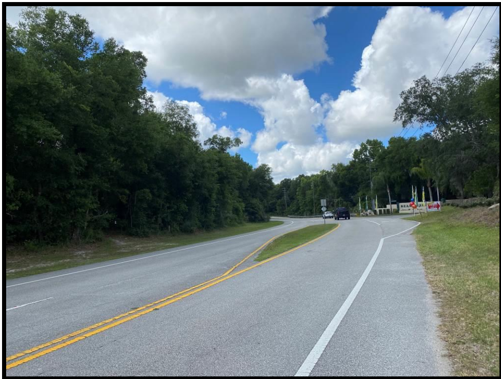
VIEW OF AIRPORT ROAD FACING EASTERLY
