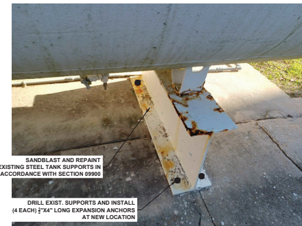
TANK SUPPORT DETAIL
