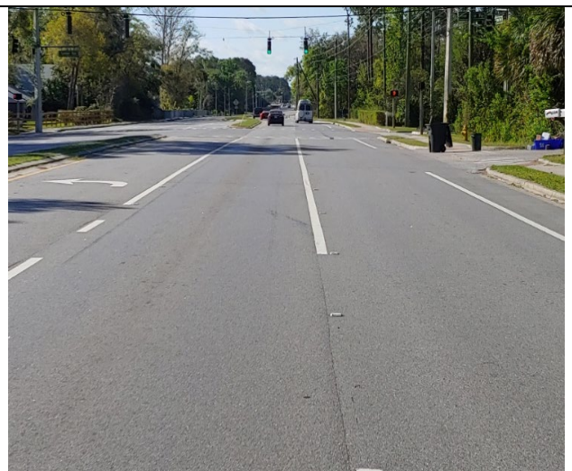
Southbound Tymber Creek Rd.
