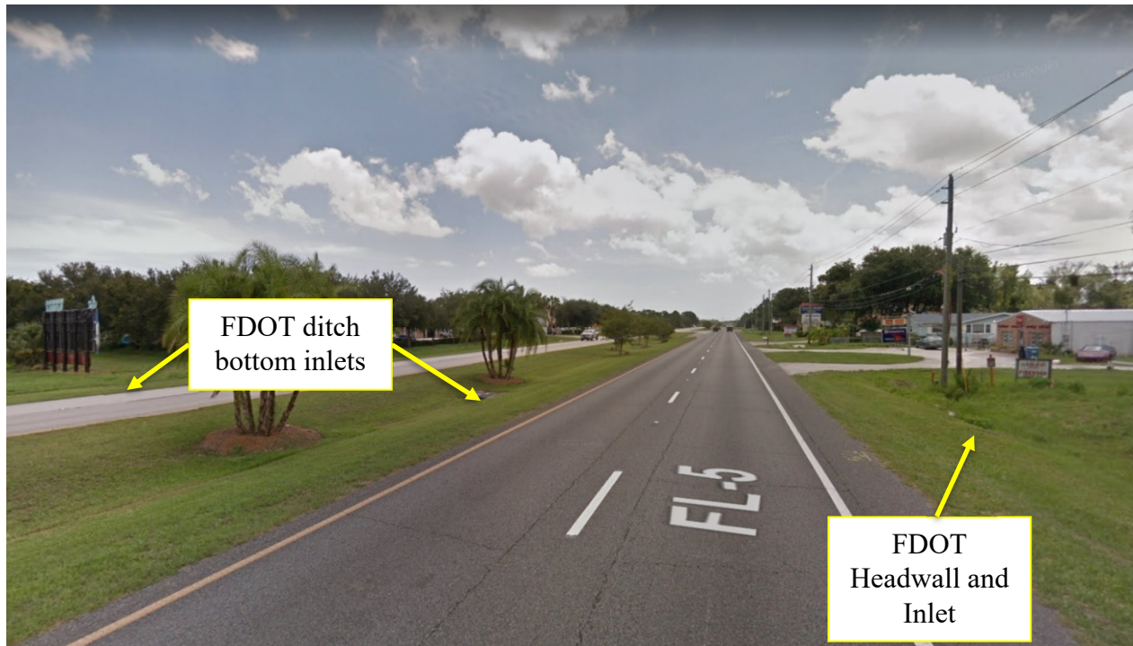
Looking south on North US Highway 1 of FDOT pipe connection to North Highway US1 Drainage swale. (Google Maps Imagery, 2019)
