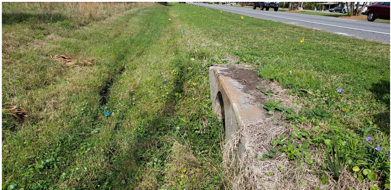
Headwall of FDOT pipe that connects the North Highway US1 Drainage swale to the FDOT pipe system. (2/19/2020)
