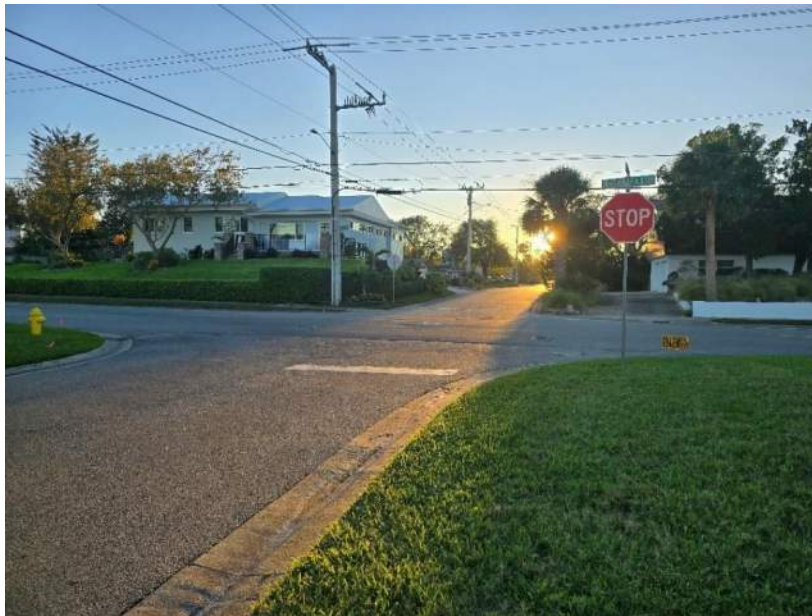
North Halifax Drive & Amsden Road intersection, facing westbound
