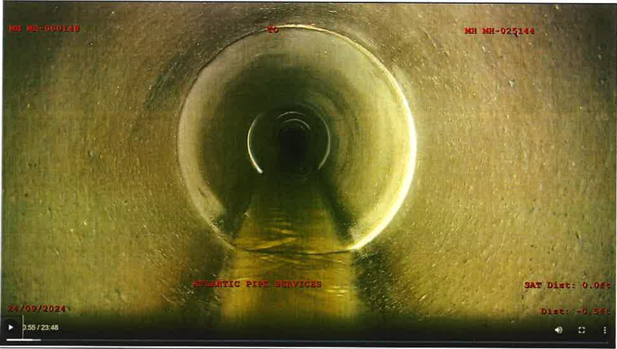
Screen Grab from a clay pipe run on Raush Camera System in 1080HD;
