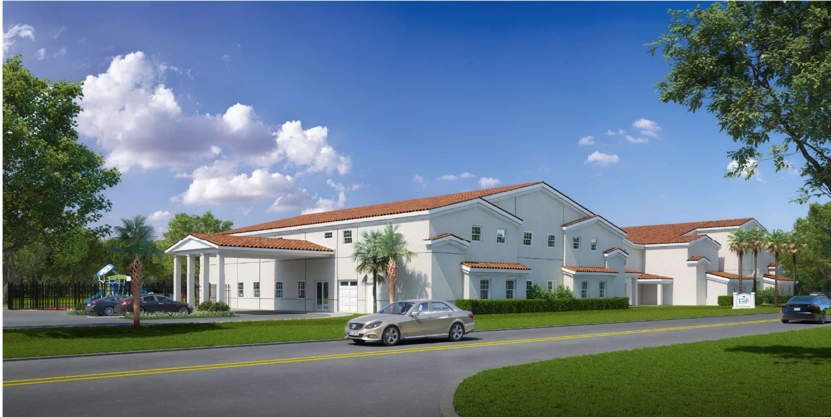
LOOKING SE FROM CORNER OF S. HALIFAX DRIVE & ARLINTON WAY
