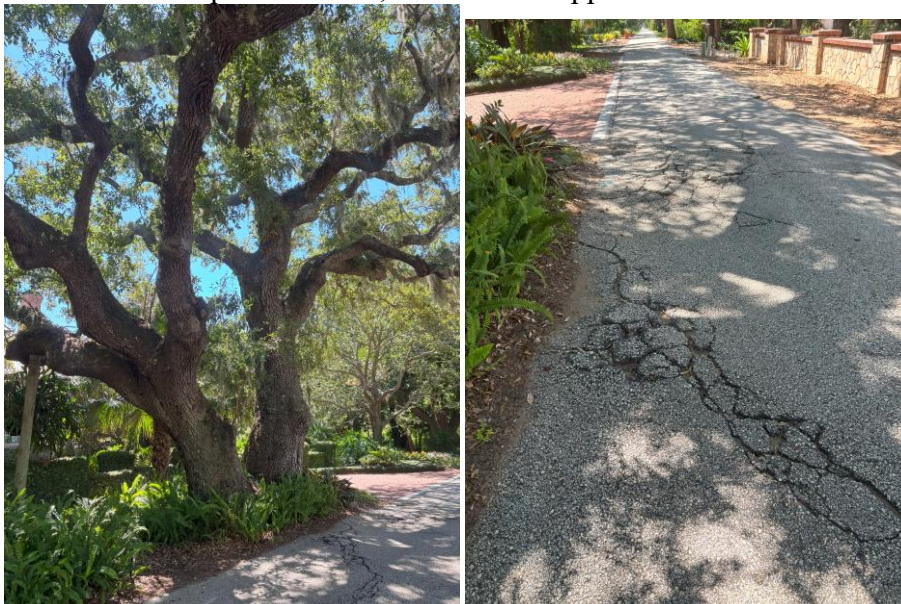
Trees #20 & #21– Riverside Dr – Asphalt is lifted, cracked and appears to be structural roots. Air Spade needed.
