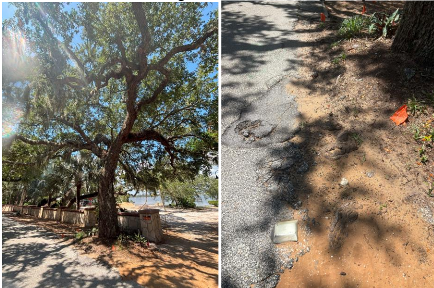
Trees #20 & #21– Riverside Dr – Asphalt is lifted, cracked and appears to be structural roots. Air Spade needed.
