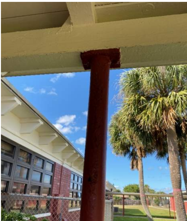
Steel Columns and Plates are Rusty and Deteriorated
