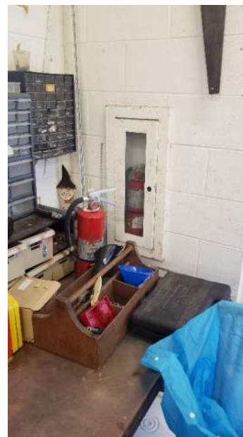
Inaccessible FE cabinet in Custodial Storage
