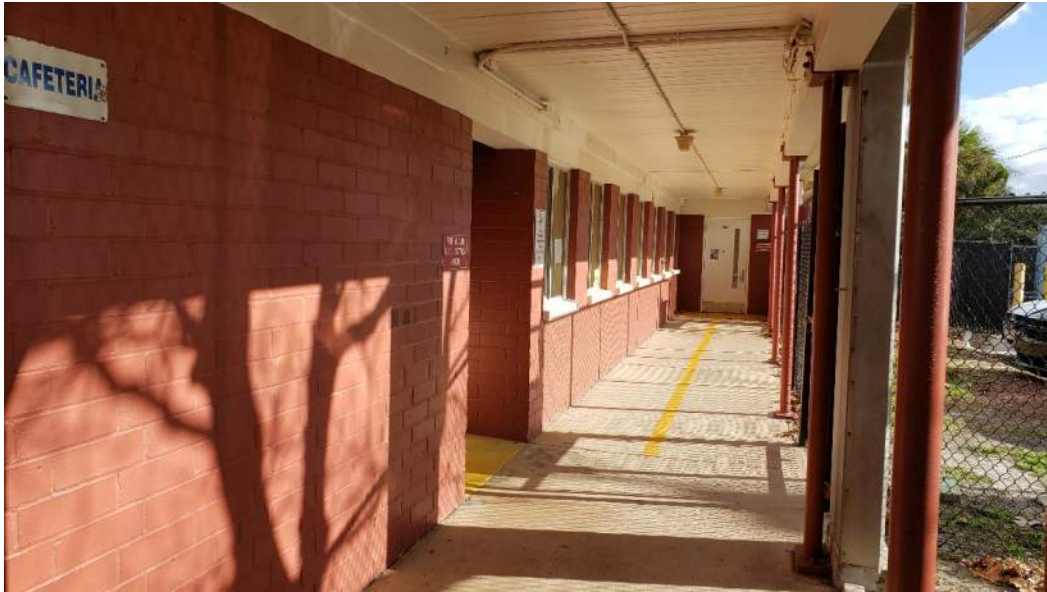
Exterior of Building
