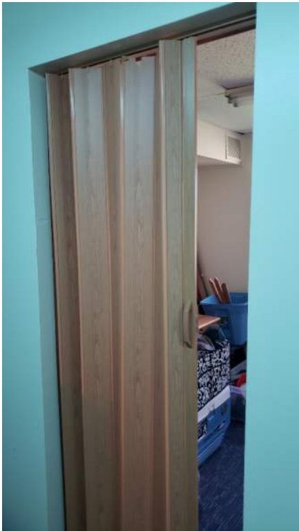
Vinyl Accordion Door to Storage
