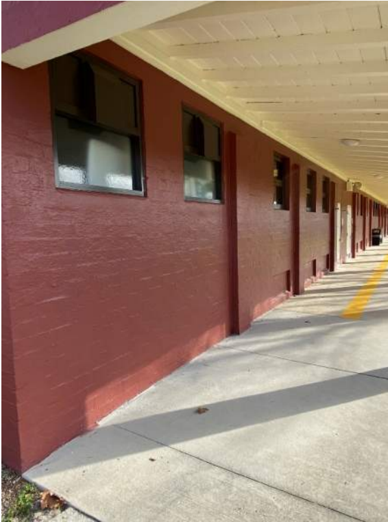
Exterior of Building 2
