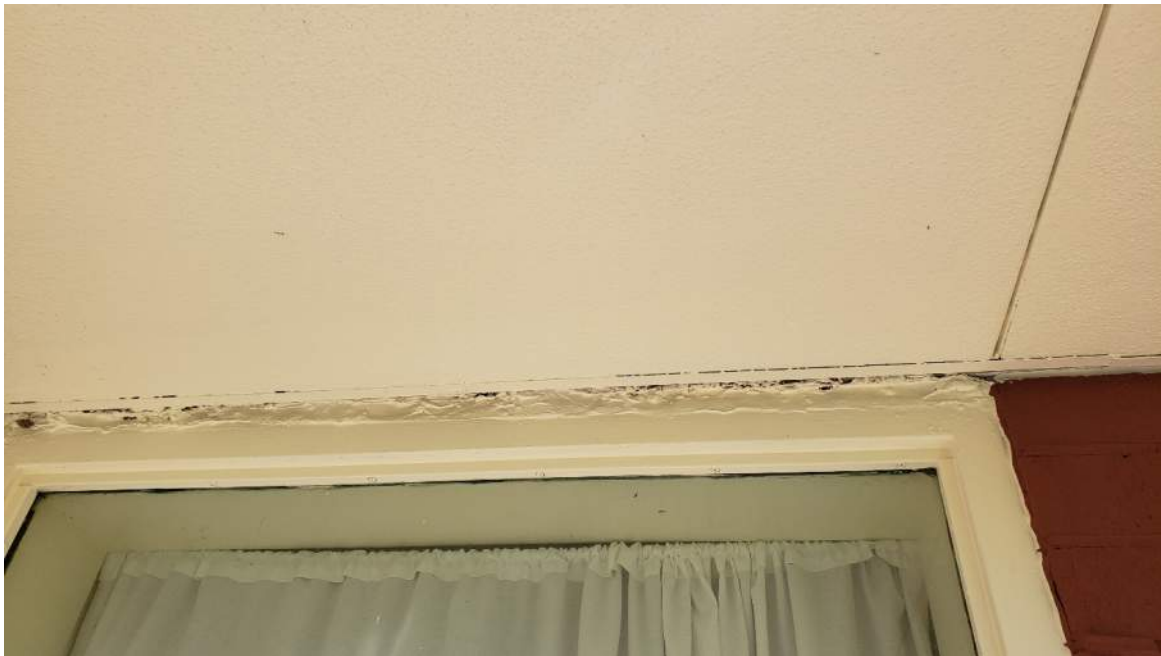
Caulking at Gaps Above Transom Windows
