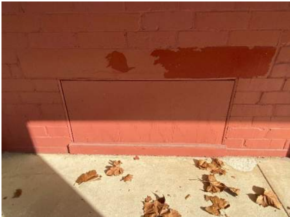
Plywood Covered Vent
