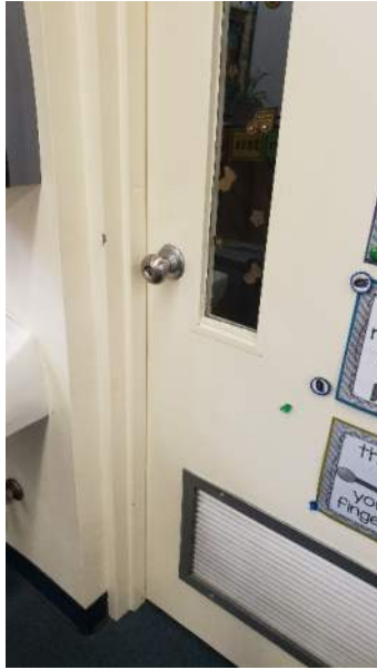
Orbital Knobs Remain on Doors
