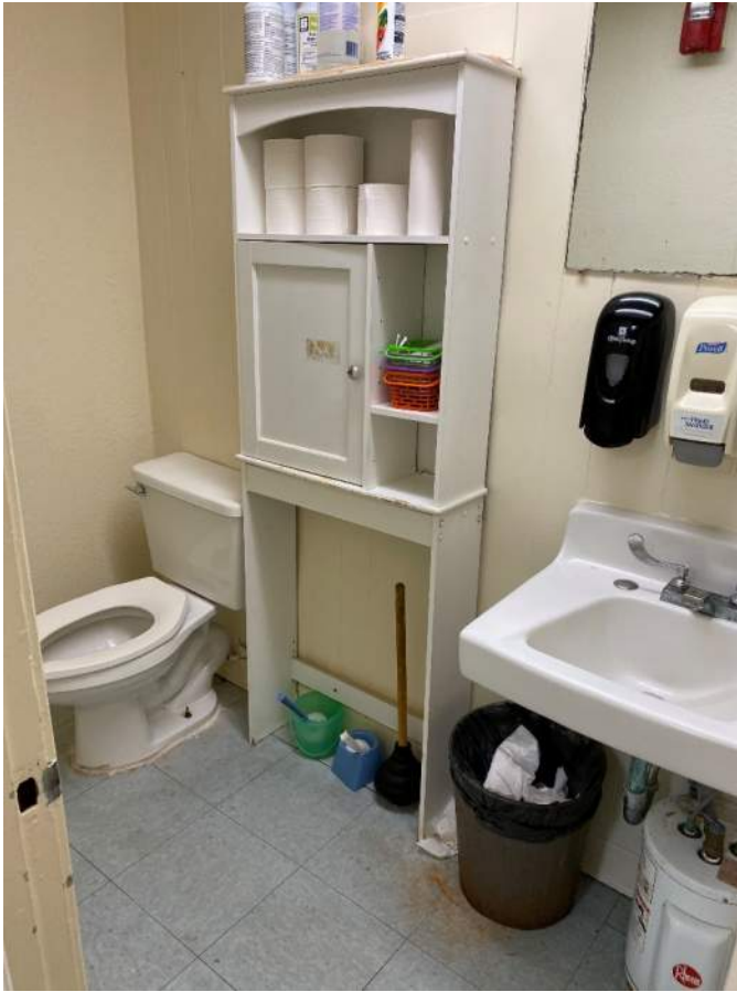
Single Restroom in Food Services Building
