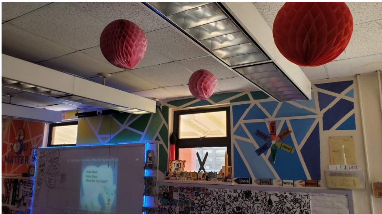
1989 Linear Pendant Light Fixture & Ceiling Replacement
